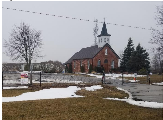
Plate 4: View of the large deciduous tree in the parking lot (visible on the left). Chain link fence along the eastern property boundary and the asphalt driveway are also visible.
