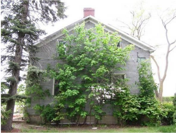
Plate 16: West elevation of the farmhouse, looking east (ASI 2010).
