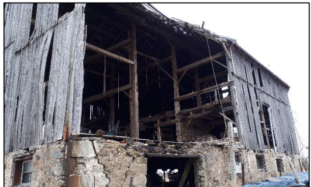
Plate 25: Interior view of the barn from exterior showing frame construction
