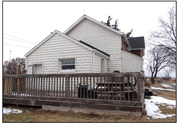
Plate 11: West elevation of original residence and one-storey rear addition
