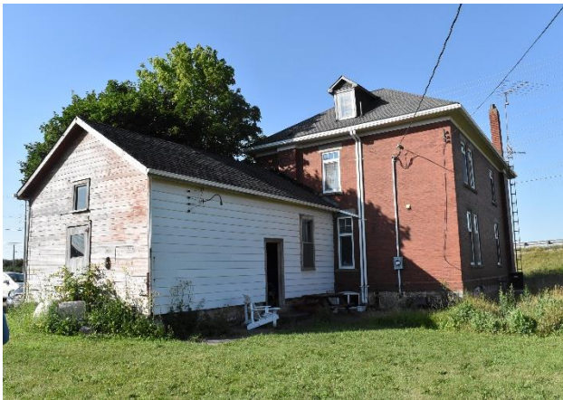
Plate 20: Single-storey, wooden frame structure at rear of house, facing west (Town of Oakville, 2018).
