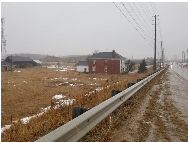
Plate 8: Embankment supporting Sixth Line, facing south.
