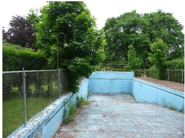
Plate 23: Concrete pool looking south (Town of Oakville 2014).
