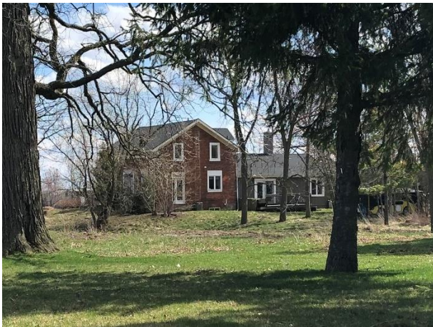
Plate 8: View of the northwest elevation (April 2020)
