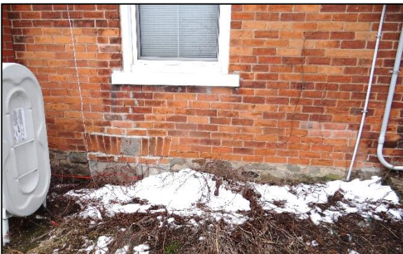
Plate 12: Stone foundation of original residence and basement window (in-filled)
