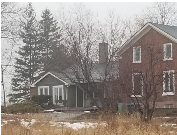
Plate 10: Detail of the board and batten rear addition and some of the brick addition (March 2020)
