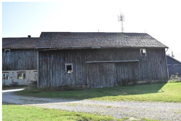
Plate 25: Driveshed, facing east (Town of Oakville, 2018).
