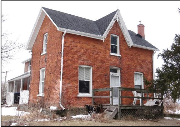
Plate 8: South (left) and east (right) elevations of original residence
