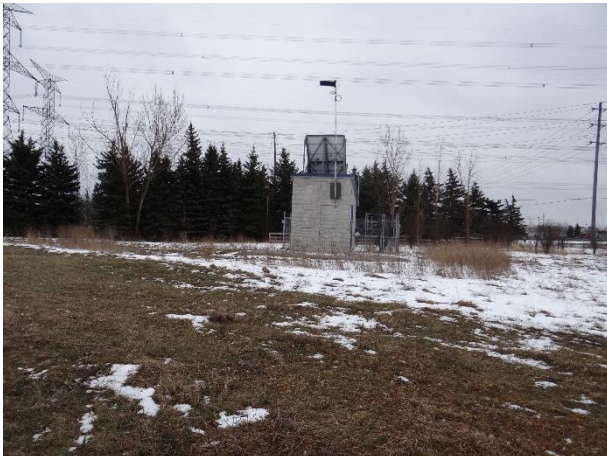
Plate 3: View of the consumers gas related building at west part of property, looking south
