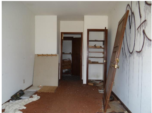
Plate 25: Former kitchen, looking north
