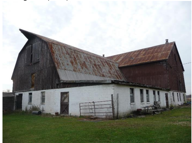
Plate 19: Barn complex showing gambrel addition (left), one-storey flat roof addition (centre) and heavy timber bank barn (right/rear) (Town of Oakville 2014).
