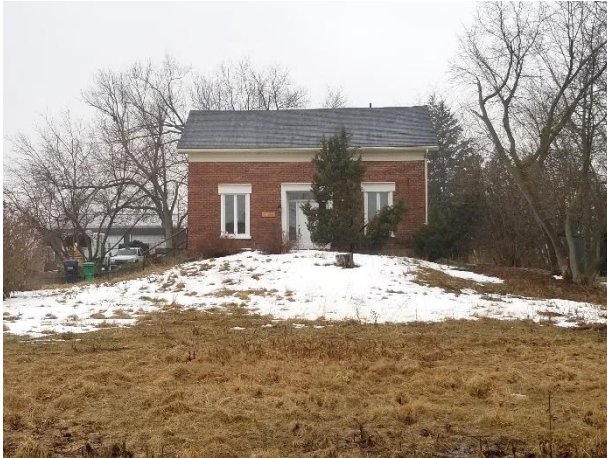
Plate 6: View of the northeastern elevation (March 2020)
