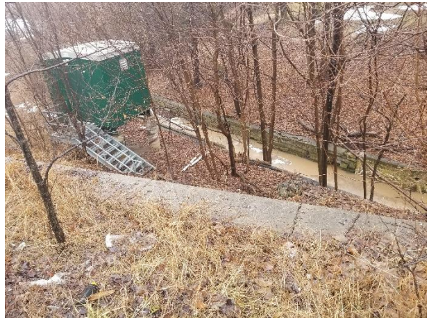
Plate 9: Stone shoring and utility structure adjacent to the creek (2020).
