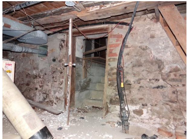
Plate 19: View of the basement looking east.
