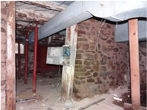
Plate 18: View of the basement looking west.
