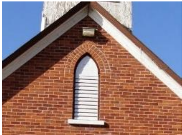
Plate 9: Detail of the ventilation window on east elevation. Date unknown (Anonymous 2019).
