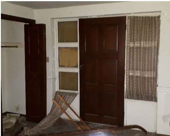
Plate 22: View of the front door from the foyer, looking west
