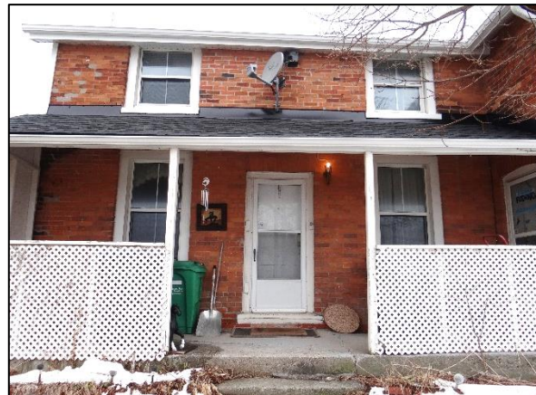
Plate 17: Detail of secondary entrance and replacement veranda on south elevation
