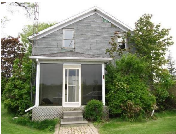
Plate 14: East elevation of the farmhouse, looking west (ASI 2010).
