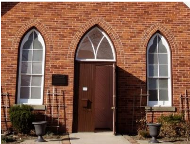
Plate 8: Detail of the entryway and windows on east elevation. Date unknown (Anonymous 2019).
