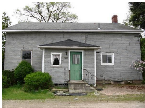
Plate 15: Rear (north) elevation of the farmhouse, looking south (ASI 2010).
