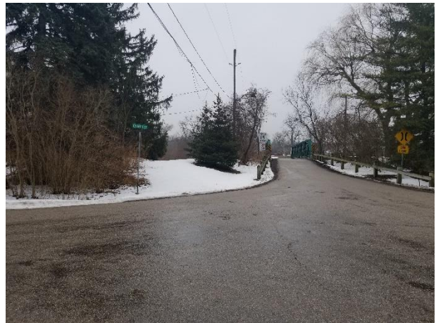
Plate 2: View of the steel pony truss bridge from the intersection of Church Street and Creditview Road.
