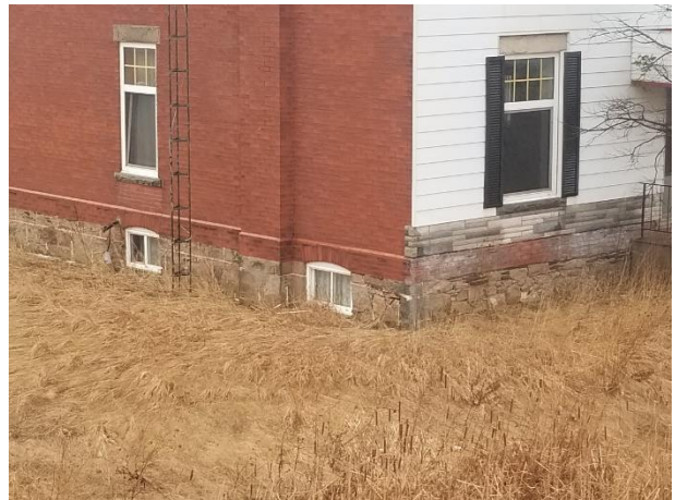
Plate 15: Stone foundation, north elevation.
