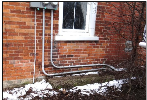
Plate 19: Detail of concrete feature along foundation and in-filled doorway (right), suggesting the location of a former veranda
