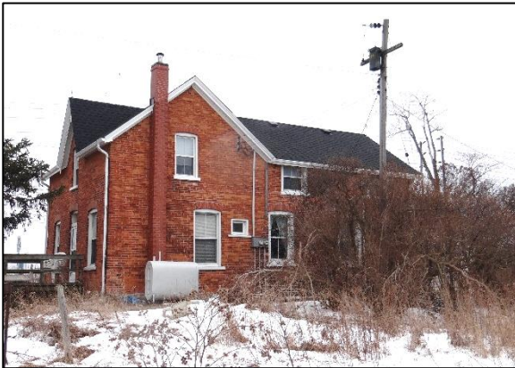
Plate 10: North elevation of original residence
