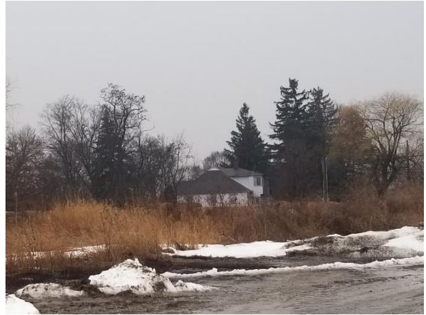
Plate 17: East elevation of twentieth-century dwelling, looking west (2020).
