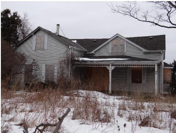
Plate 6: West elevation, log house portion is on the left
