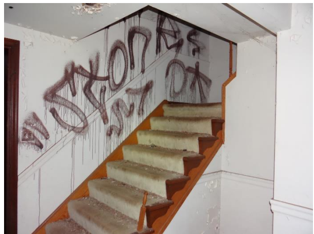
Plate 21: Staircase to second floor, from main floor foyer
